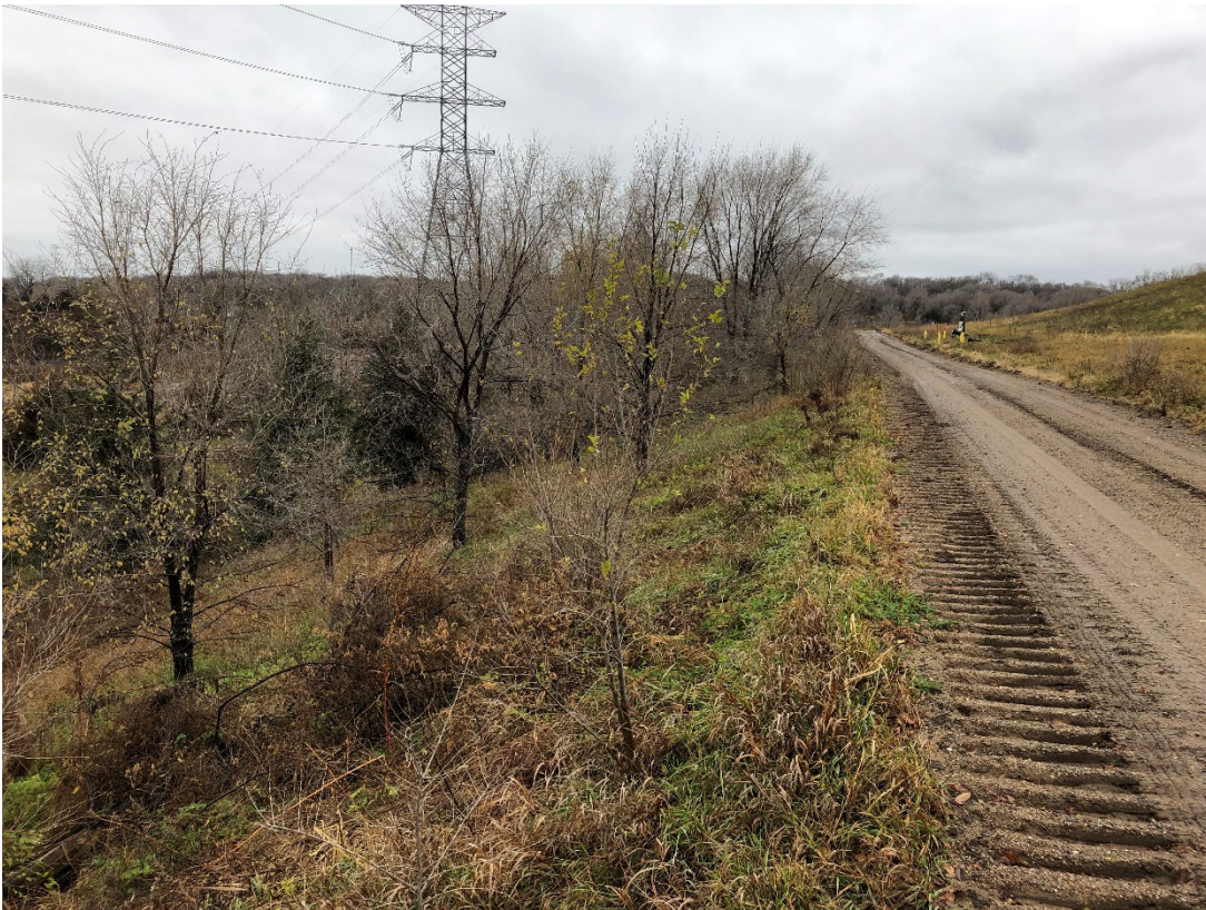
Photo 30: Location 12 – Looking Northwest, Cell 2B Southwestern Berm
