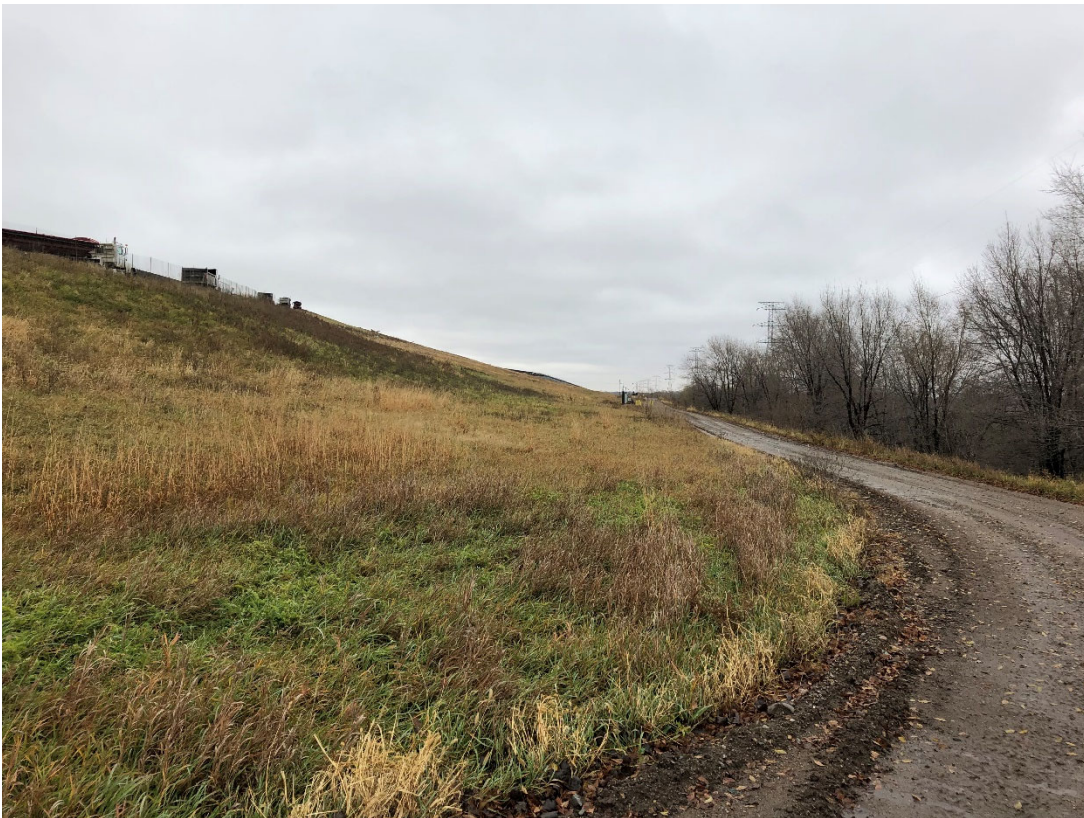
Photo 36: Location 14 – Looking Southeast, Cell 2A Southwestern Waste Slope
