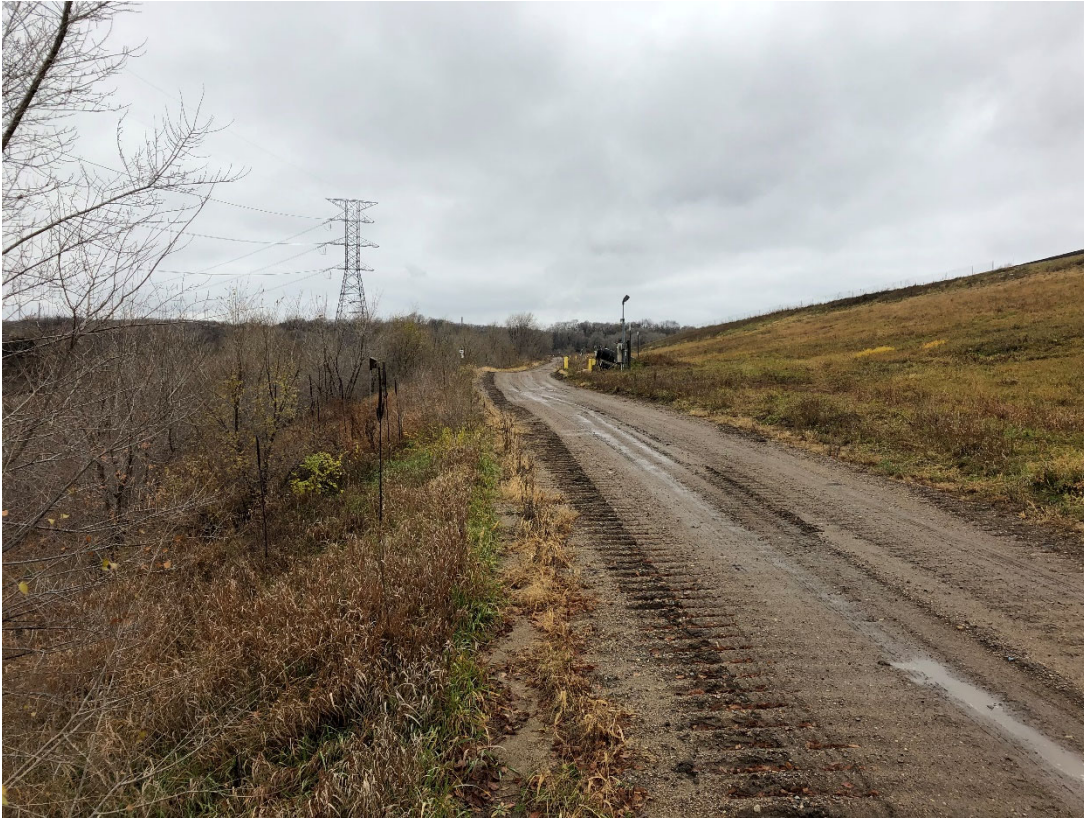
Photo 23: Location 10 – Looking Northwest, Cell 2C Cell 2C Southwestern Berm
