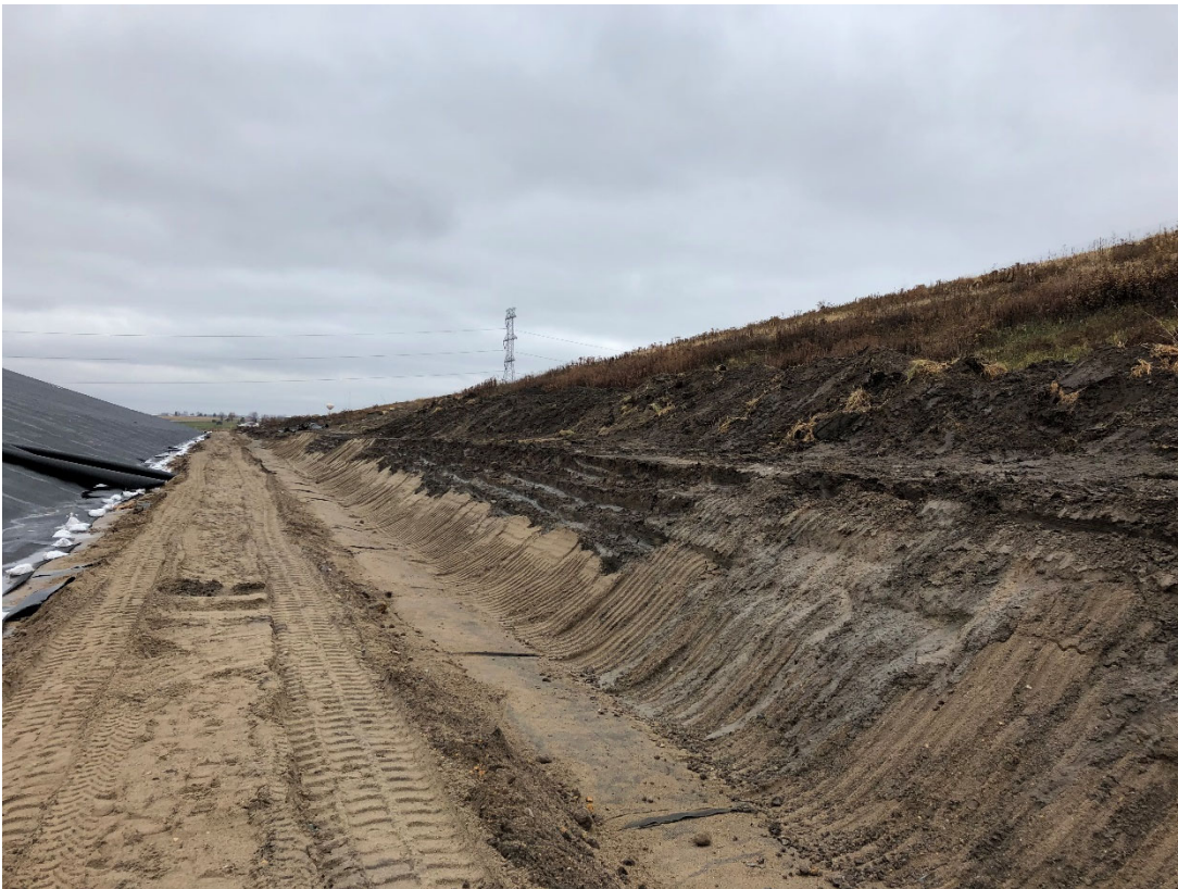
Photo 14: Location 6 – Looking Southwest, Southeastern Slope, Anchor Trench & New Liner Construction
