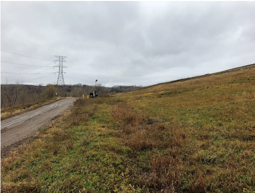
Photo 22: Location 10 – Looking Northwest, Cell 2C Southwestern Slope, Anchor Trench, and Road
