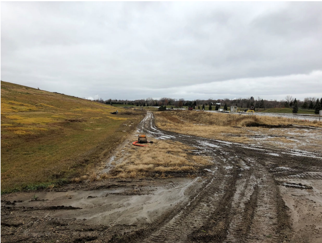
Photo 6: Location 3 – Looking Northwest, Phase 3A Anchor Trench and Northeastern Waste Slope
