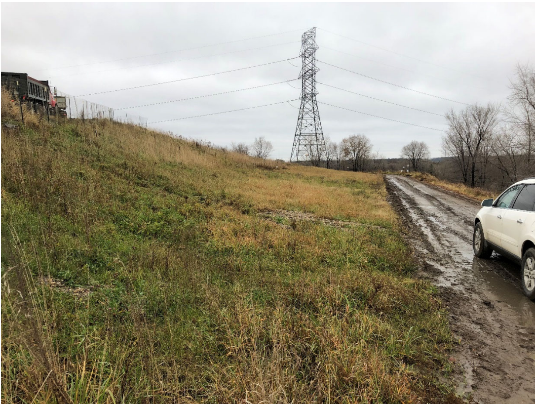
Photo 40: Location 15 – Looking Southwest, Cell 2A Northwest Waste Slope and Anchor Trench
