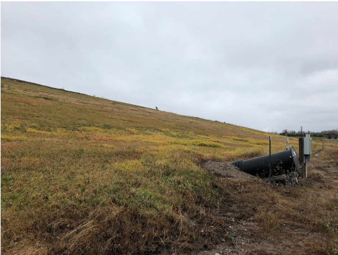
Photo 4: Location 2 – Looking Northwest, Cell 3 Anchor Trench and Waste Slope
