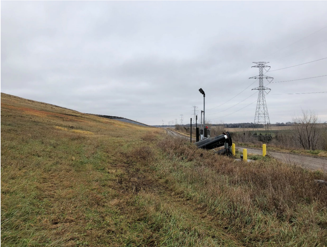
Photo 25: Location 11 – Looking Southwest, Cell 2C Southwestern Waste Slope and Anchor Trench
