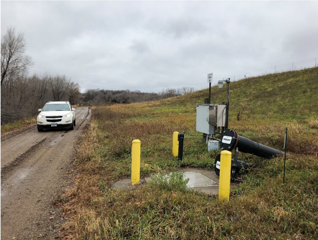
Photo 33: Location 13 – Looking Northwest, Cell 2A Southwestern Waste Slope and Perimeter Road
