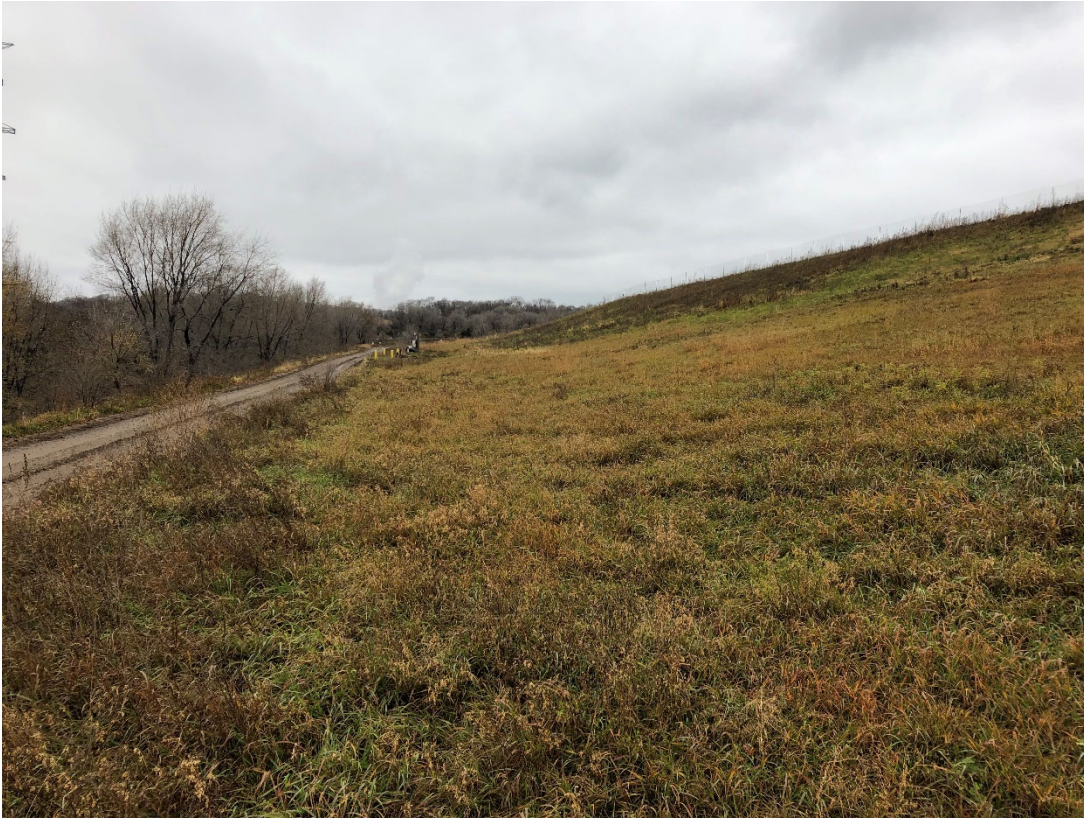
Photo 29: Location 12 – Looking Northwest, Cell 2B Southwestern Waste Slope and Anchor Trench
