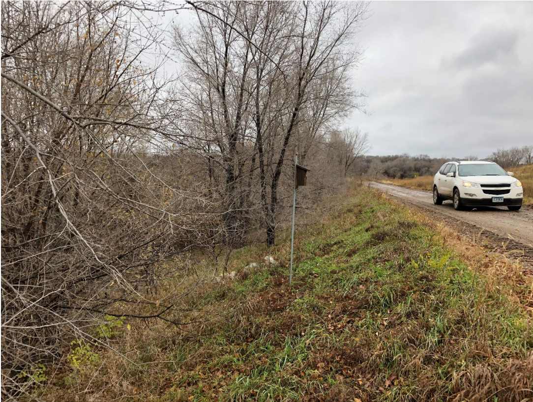
Photo 31: Location 13 – Looking Northwest, Cell 2A Southwestern Berm
