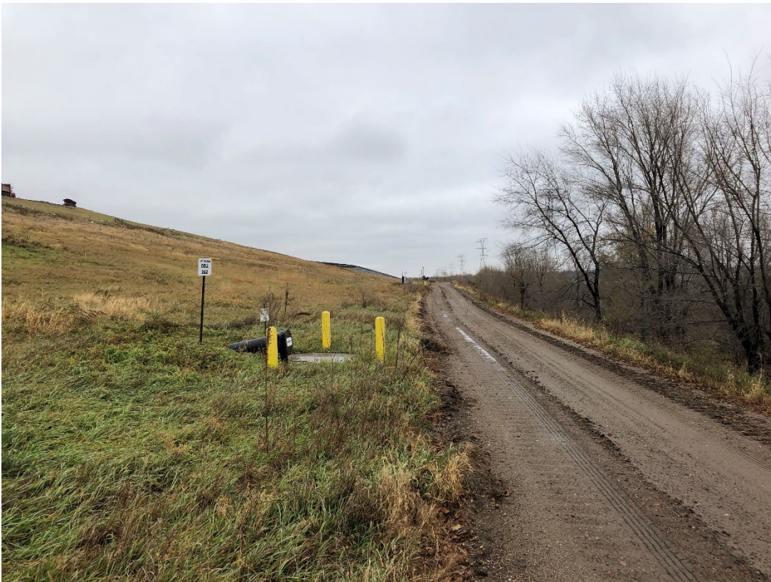
Photo 34: Location 13 – Looking Southeast, Cell 2B Southwestern Waste Slope and Perimeter Road
