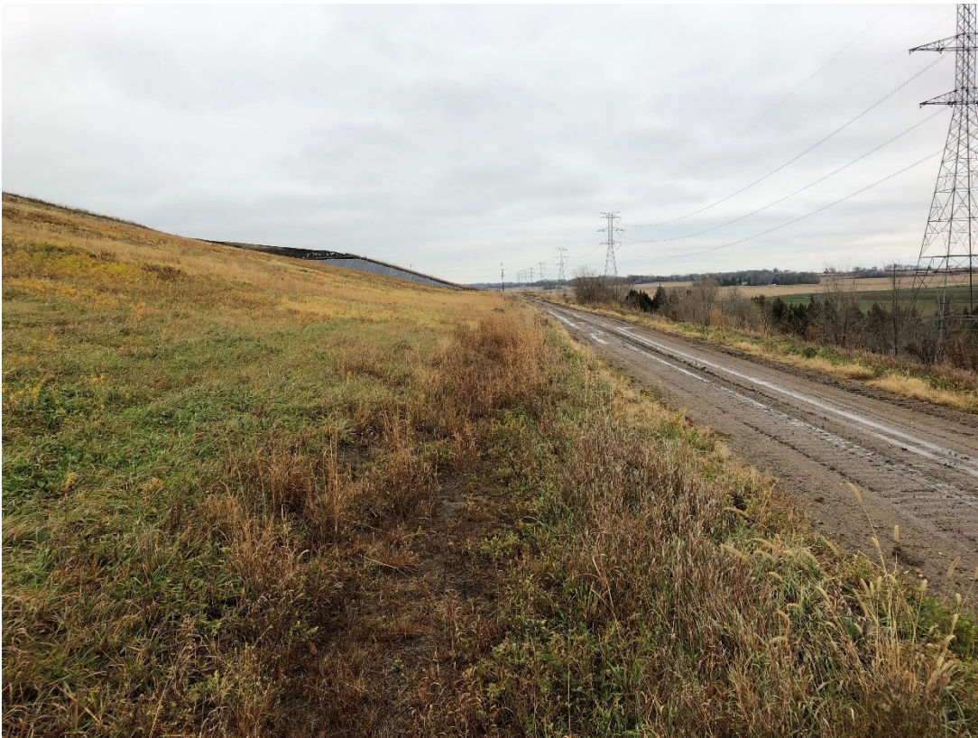
Photo 20: Location 10 – Looking Southeast, Cell 2D Southwestern Slope, Anchor Trench, and Road
