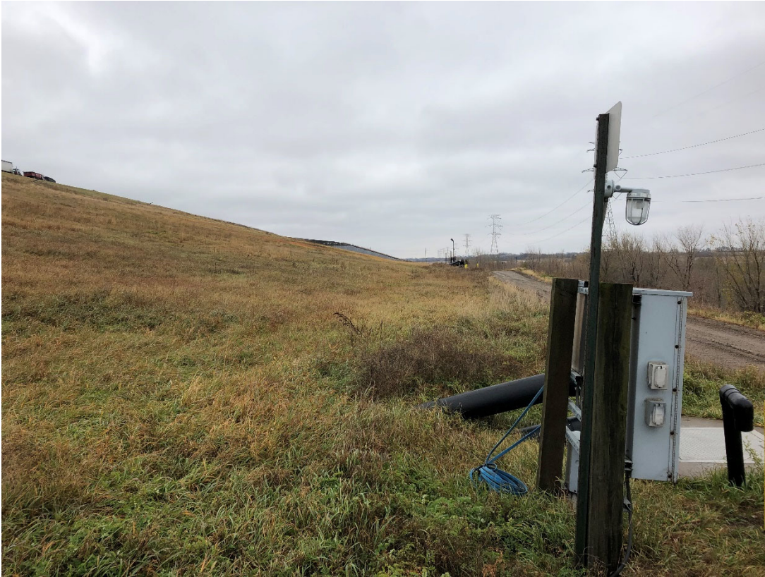
Photo 27: Location 12 – Looking Southeast, Cell 2C Southwestern Waste Slope and Anchor Trench
