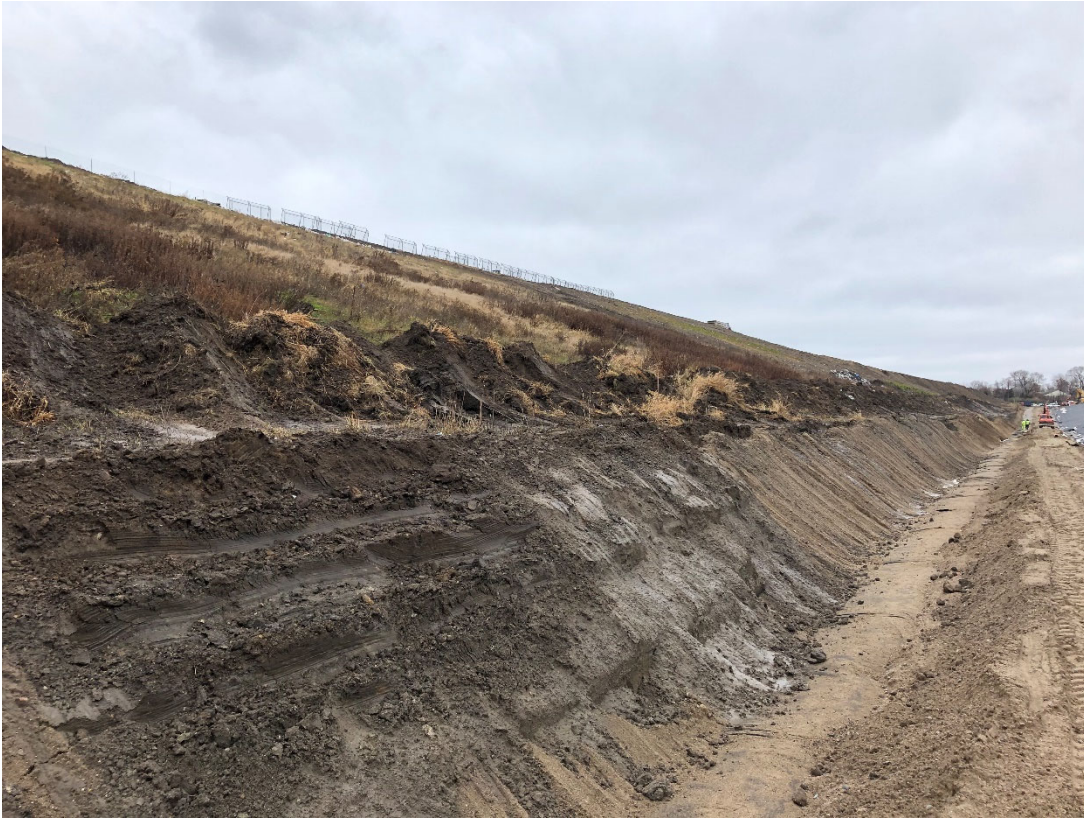
Photo 13: Location 6 – Looking Northeast, Southeastern Slope, Anchor Trench & New Liner Construction
