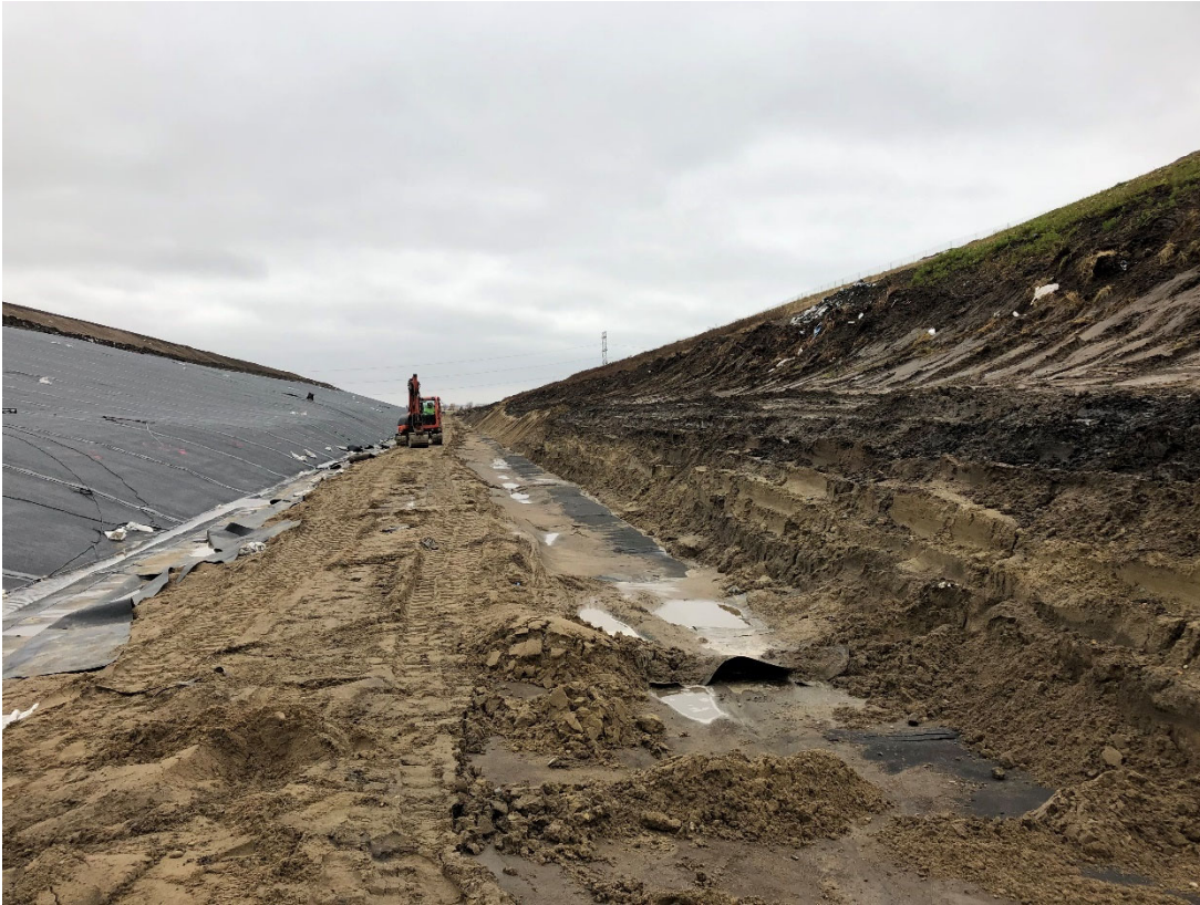
Photo 9: Location 4 – Looking Southwest, Southeastern Slope, Anchor Trench & New Liner Construction
