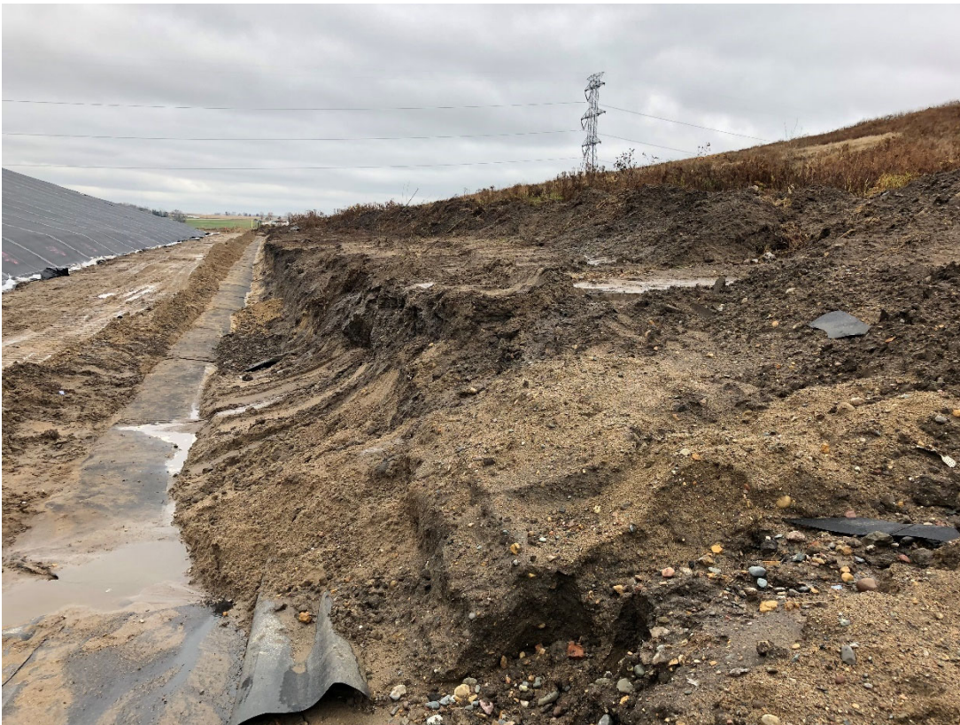
Photo 16: Location 8 – Looking Southwest, Southeastern Slope, Anchor Trench & New Liner Construction
