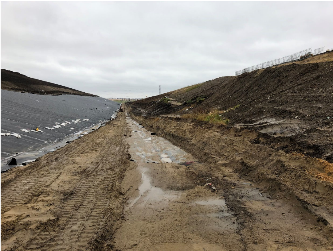
Photo 8: Location 3 – Looking Southwest, Southeastern Slope, Anchor Trench & New Liner Construction
