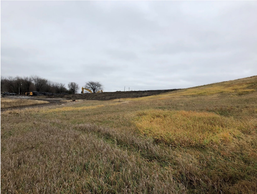
Photo 5: Location 2 – Looking Southeast, Phase 3A Anchor Trench and Northeastern Waste Slope
