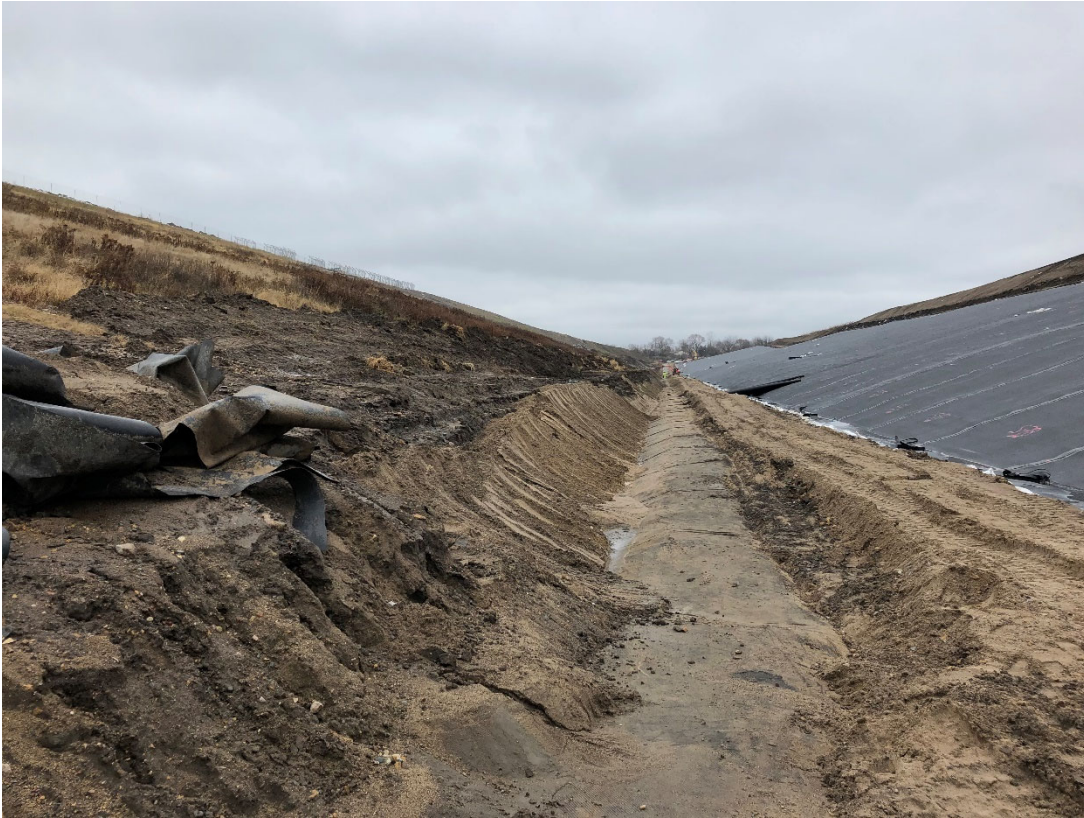
Photo 15: Location 8 – Looking Northeast, Southeastern Slope, Anchor Trench & New Liner Construction
