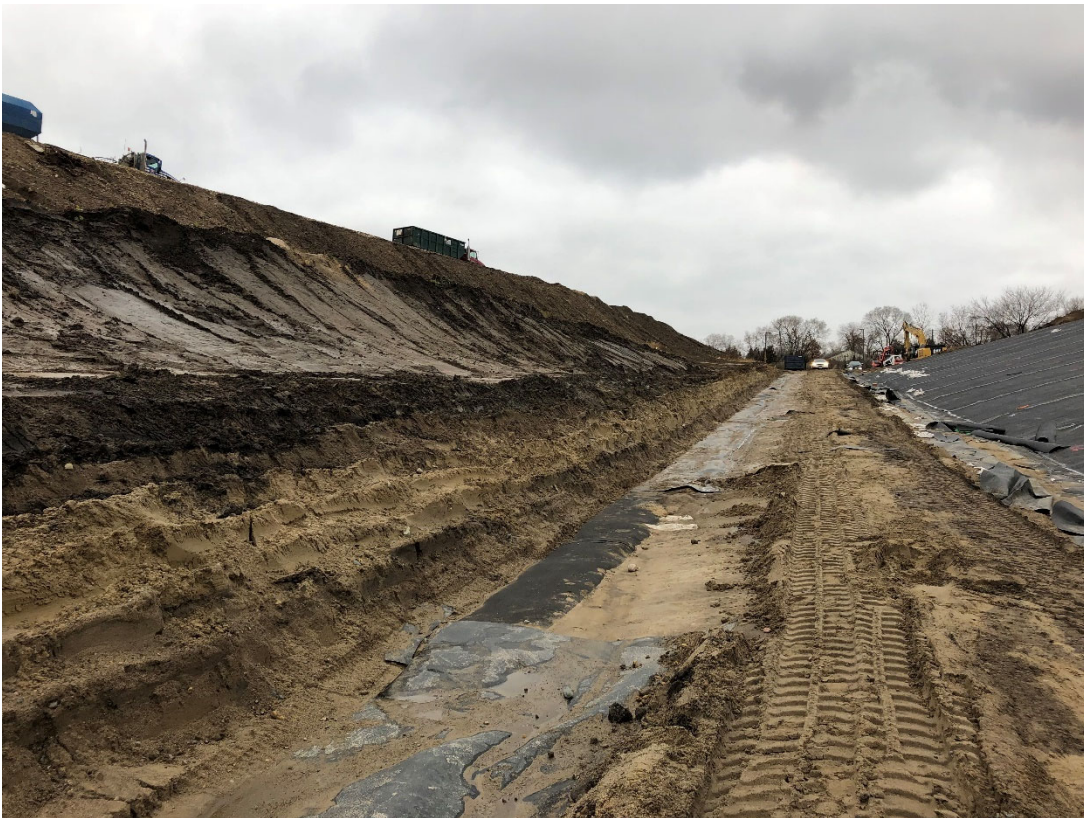
Photo 10: Location 4 – Looking Northeast, Southeastern Slope, Anchor Trench & New Liner Construction
