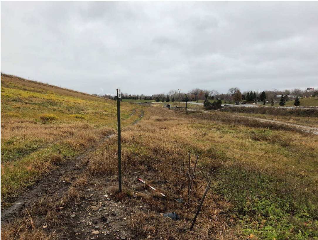
Photo 2: Location 1 – Looking Northwest, Cell 3 Berm
