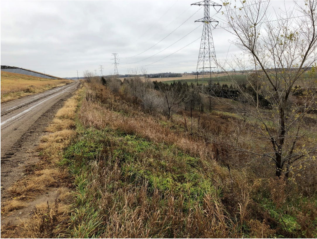
Photo 21: Location 10 – Looking Southeast, Cell 2D Berm
