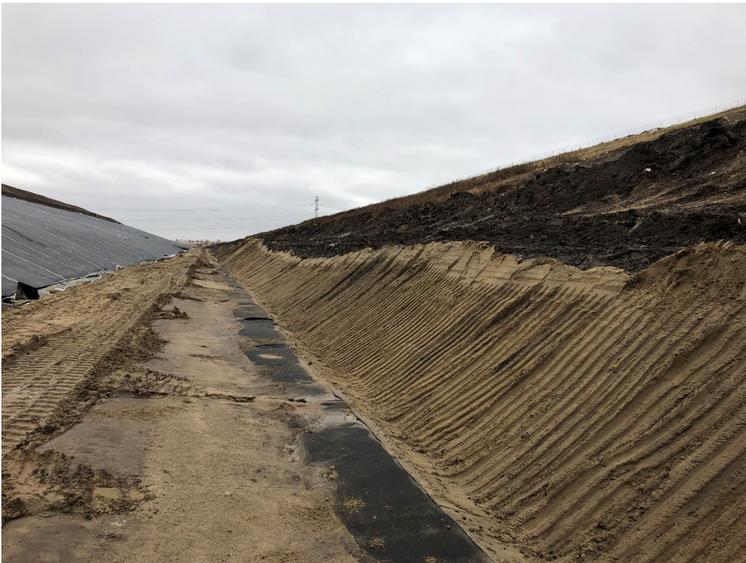
Photo 12: Location 5 – Looking Southwest, Southeastern Slope, Anchor Trench & New Liner Construction
