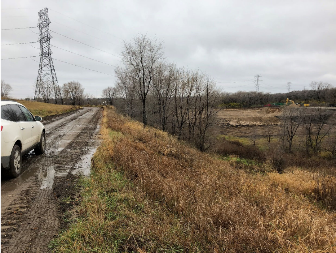
Photo 39: Location 15 – Looking Southwest, Cell 2A Northwestern Berm
