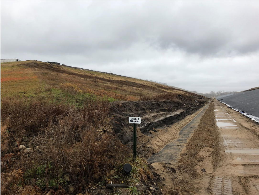
Photo 17: Location 9 – Looking Northeast, Southeastern Slope, Anchor Trench & New Liner Construction
