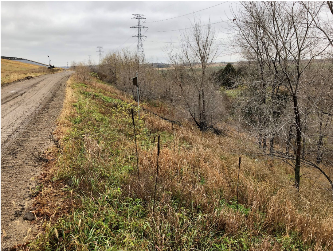
Photo 28: Location 12 – Looking Southeast, Cell 2C Southwestern Berm
