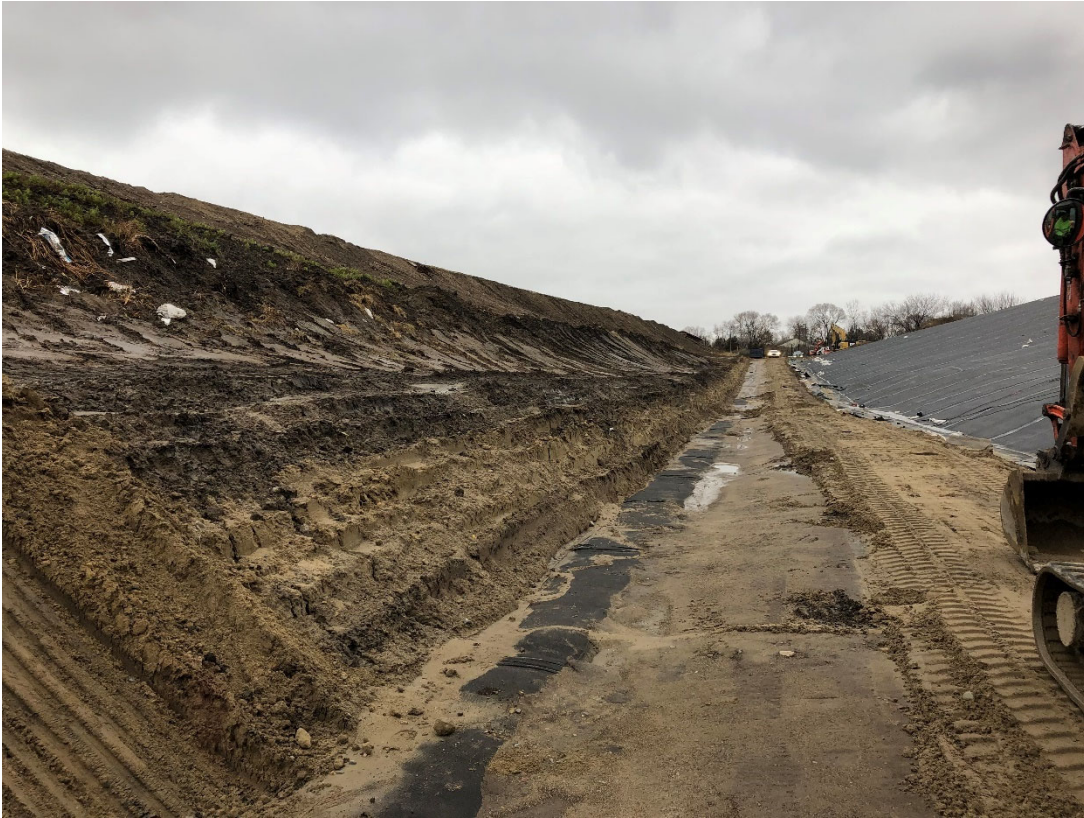
Photo 11: Location 5 – Looking Northeast, Southeastern Slope, Anchor Trench & New Liner Construction
