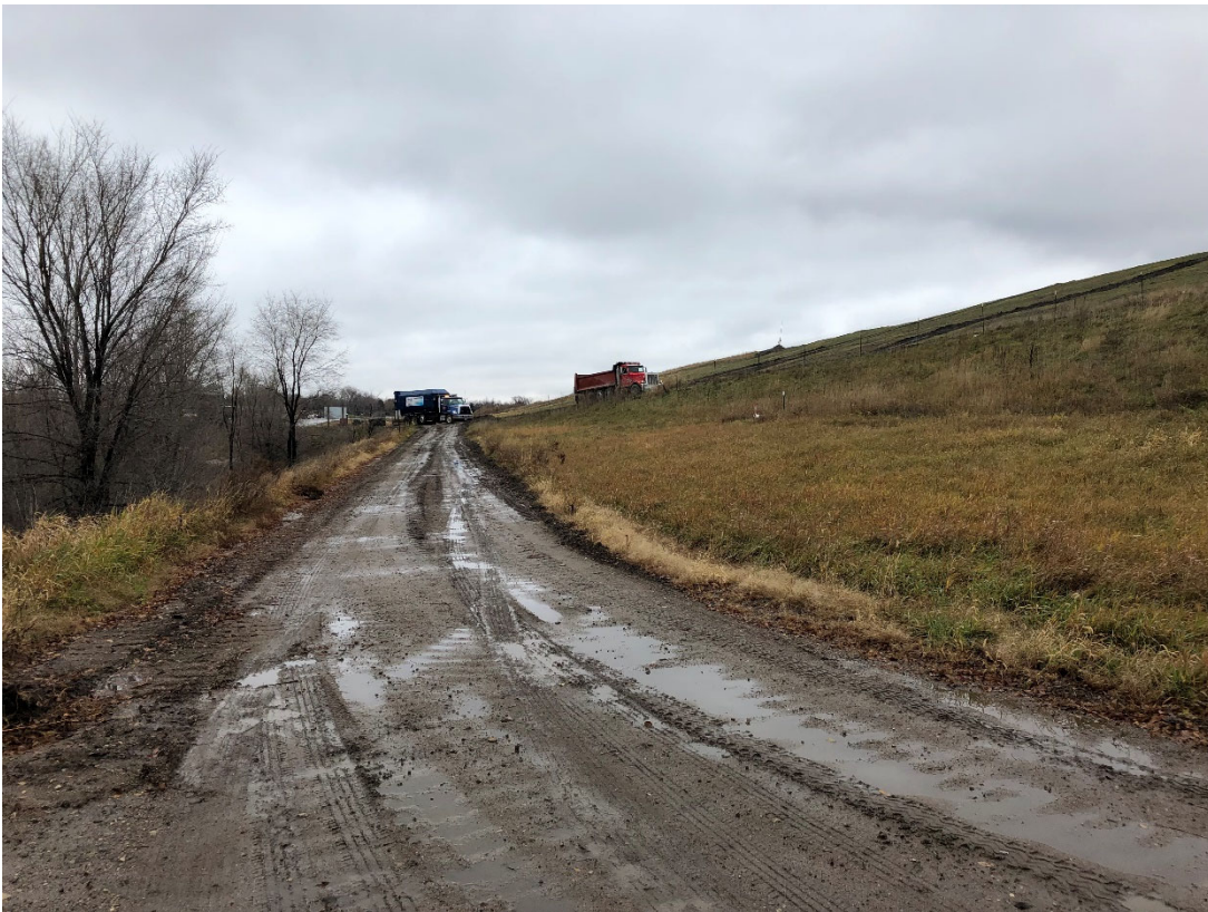
Photo 38: Location 14 – Looking Northeast, Cell 2A Northwestern Perimeter Road and Anchor Trench
